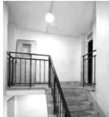
photo of stairwell with LED fitting
