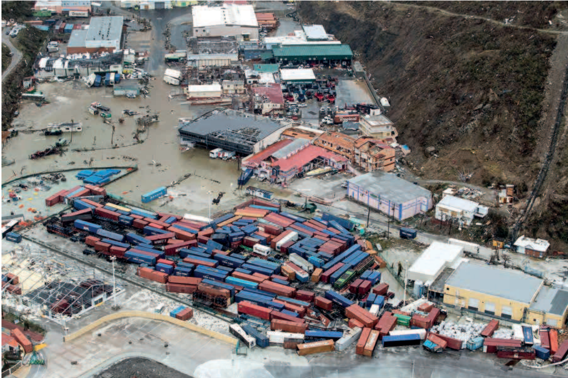
Photo: Overturned shipping containers in Sint Maarten
